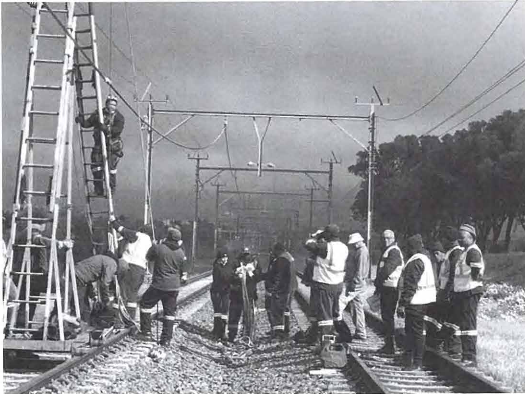
Workers repairing the rail tracks on Friday. (Photo: Tariro Washinjira)
